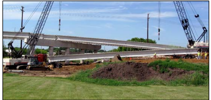
Project under construction
