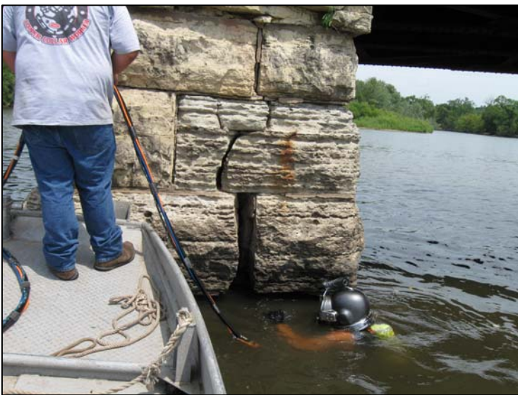
Investigations to the Cedar River Rail-Trail Bridge in Summer, 2008
