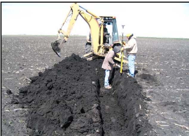
WHKS survey crew take measurements during trenching.
