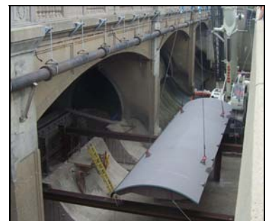
Delivery and installation of the first of five gates for the dam.
