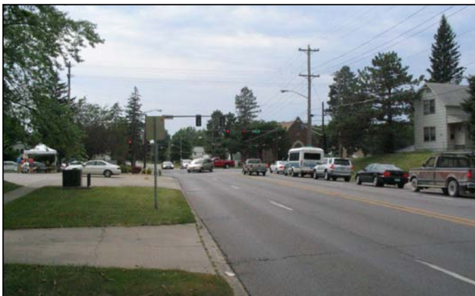
Traffic signal improvements were involved in the work.
