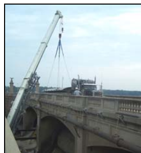
Delivery and installation of the first of five gates for the dam.
