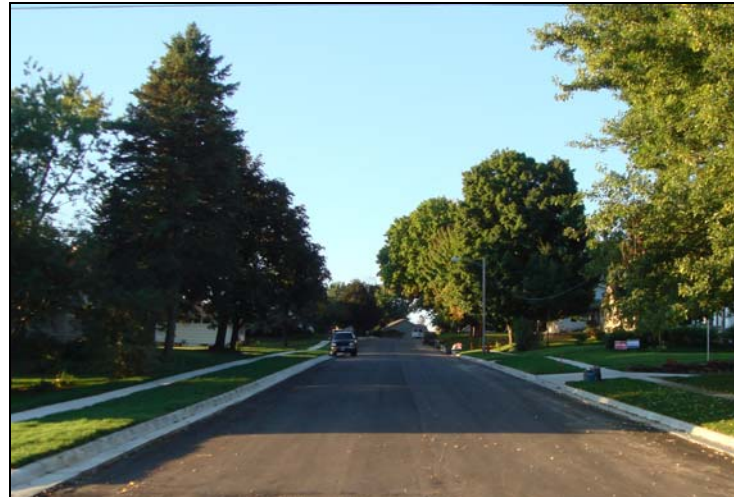
The completed Warren Avenue Reconstruction project.
