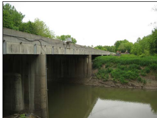
Existing bridge carrying IL 61 over the Lamoine River.
