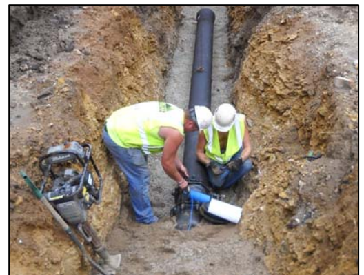
Utility replacements posed challenges.
