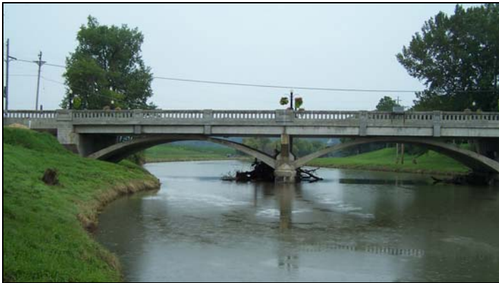
Existing IL 84 Bridge in Hanover, Illinois
