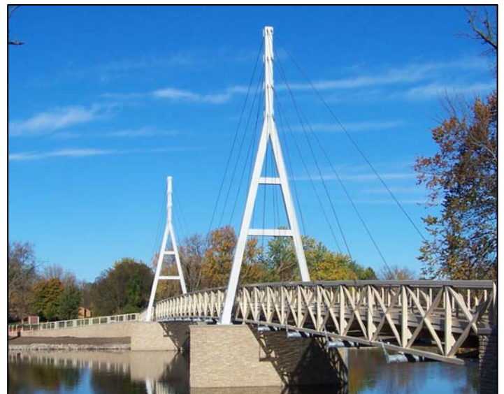
The prefabricated cable-stayed bridge option was the most economical solution for the City's desire to have a cable structure that could incorporate aesthetic treatments that are unique to the community.
