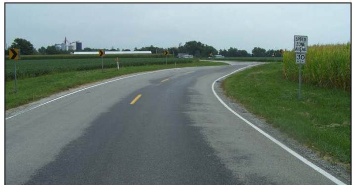
The existing horizontal and vertical alignments were improved to meet a 55 MPH design speed.
