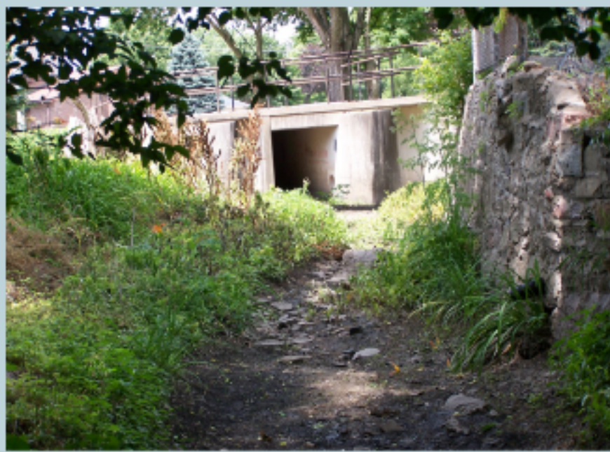
A view of the Dry Run Creek Channel before construction
