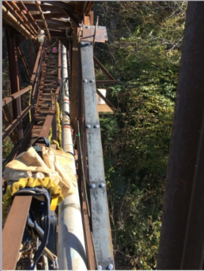
Typical Truss Diagonal Repair
