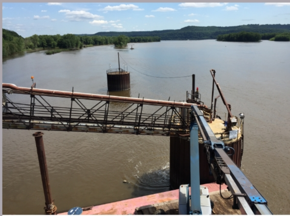
Overall Barge Loading Facility
