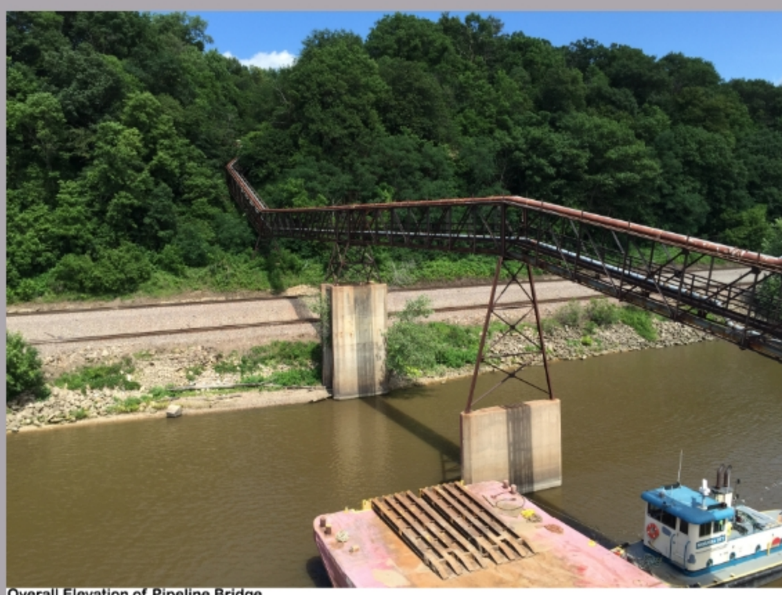
Overall Elevation of Pipeline Bridge
