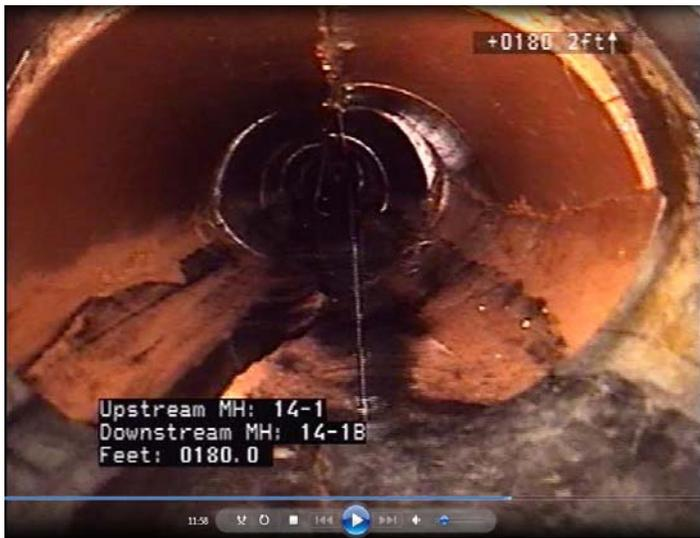
*Infiltration leaks into a trunk line sanitary sewer pipe in imminent risk of collapse near Cheslea Creek, Mason City, Iowa. This pipe and other similar pipes were repaired during the project.*
