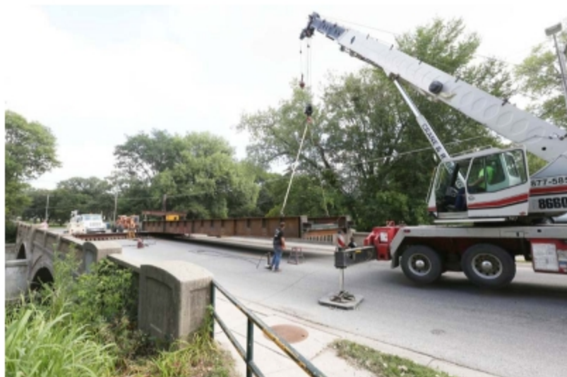
Moving contractor constructing the "bridge over the bridge"
