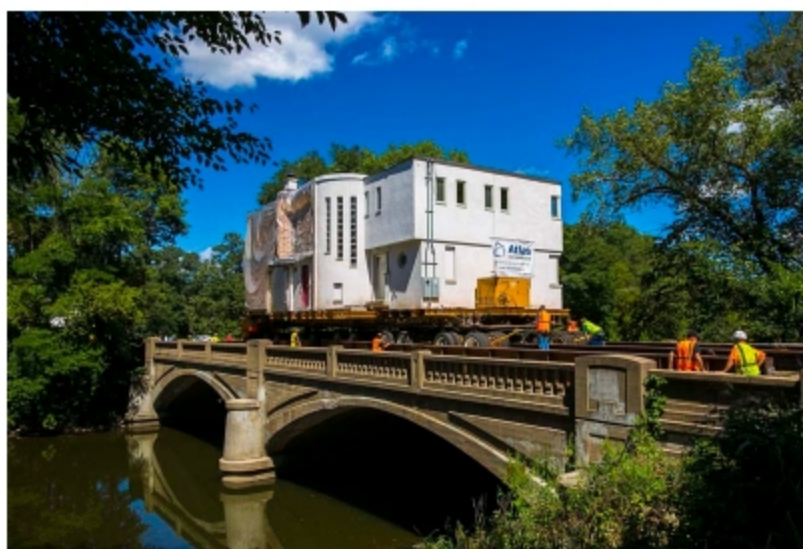
280-ton section of the Egloff House as it rolls along the "bridge over the bridge"
