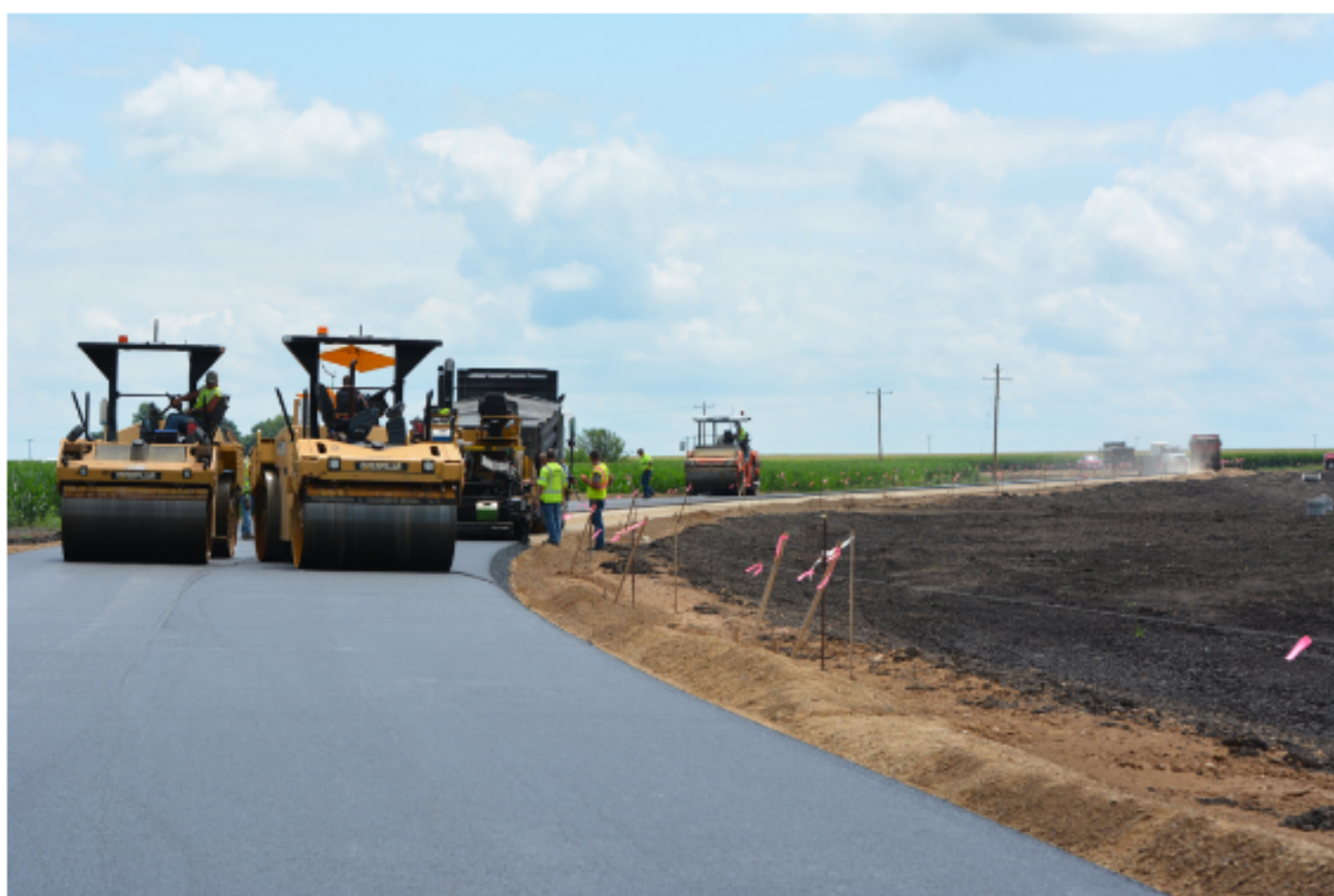
Construction of CH 30
