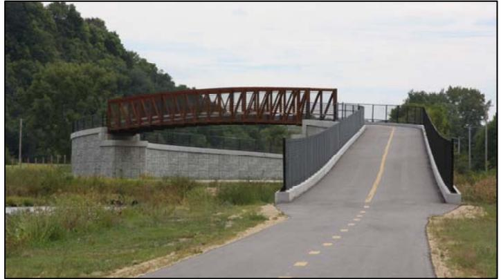
*Use of bridge abutment spread footings on MSE embankments is a unique and innovative practice in Iowa.*
