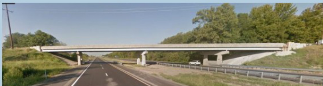
View of Baumann Road Bridge from I-70
